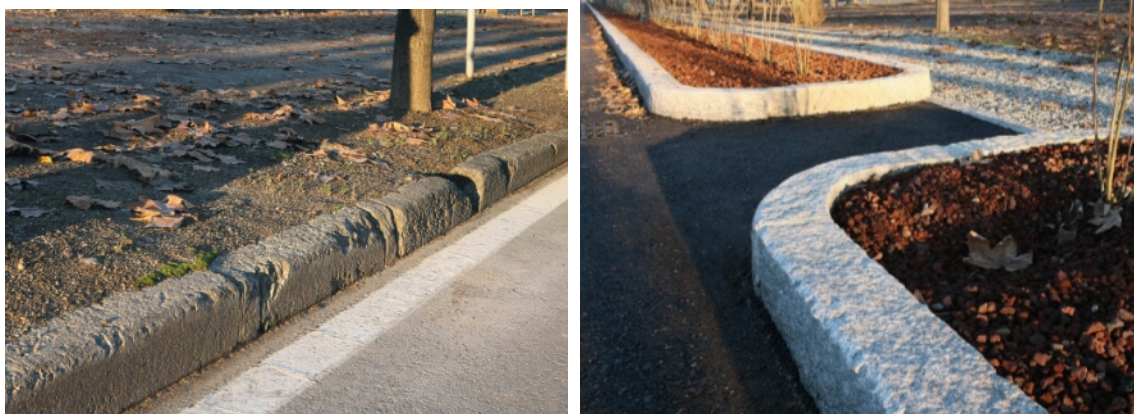
Cordoli in cemento usurati e cordoli in granito
